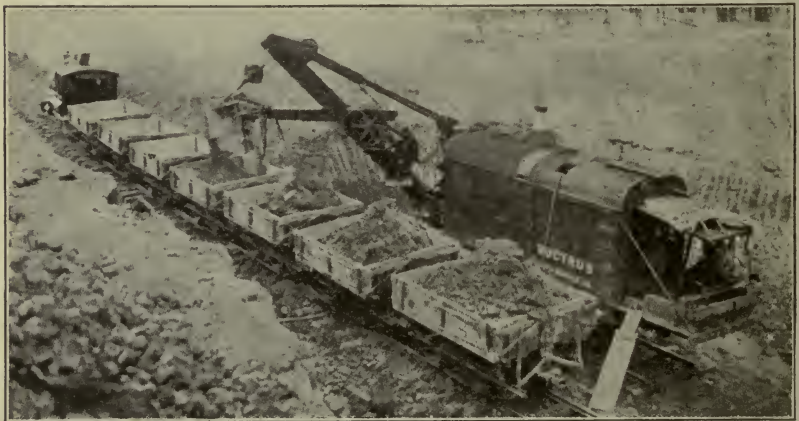
Fig. 18. Bucyrus Shovel Filling Dump Cars with Clay
